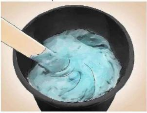
5- Wait for 20min (initial set) then, avoiding excessive water, wipe the complete area thoroughly with a damp sponge to obtain a smoother joint.
